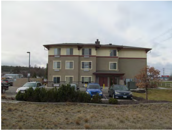
Photo #13 View of the Appleway Court Apartments on the northern adjoining property to the west.
